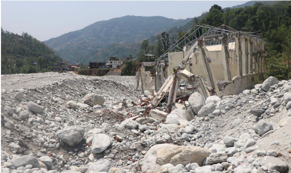
Aftermath of the flood and debris flow in Melamchi in June 2021, (Image: Yutshu Shrestha)
